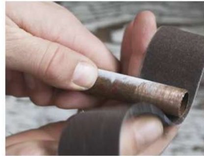
Diagram 2 showing correct sanding direction
